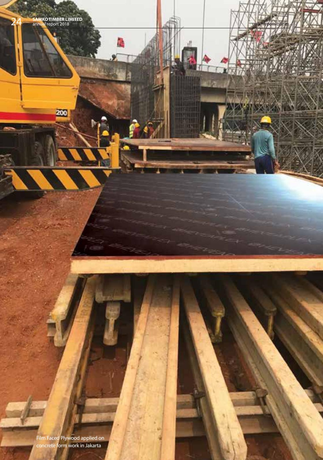
Film Faced Plywood applied on
